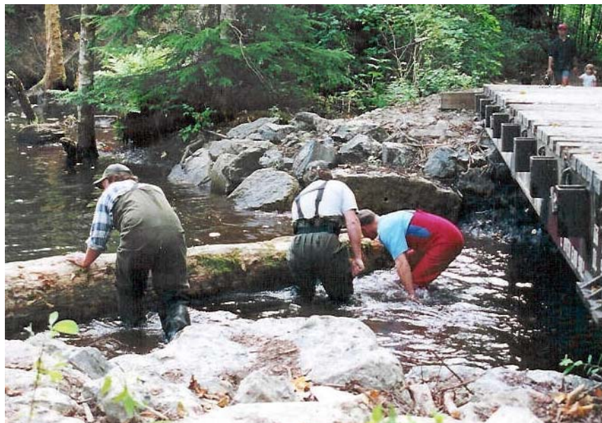
Stream enhancement by the Squamish Streamkeepers: building a "beaver baffle" on the Little Stawamus River
