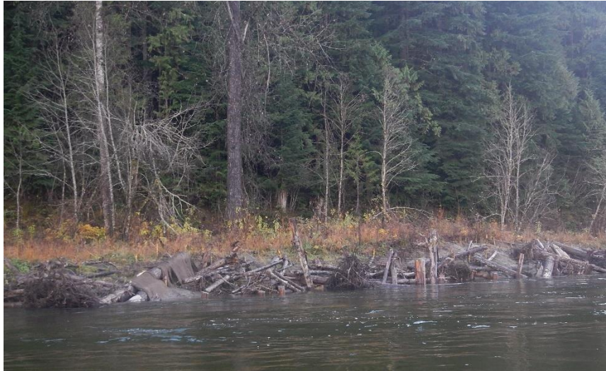
Large woody debris revetment and bank stabilization
