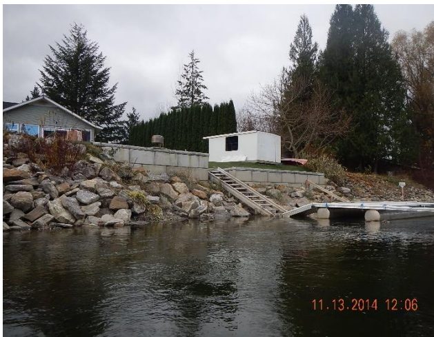
Rip rap and Bank Stabilization
