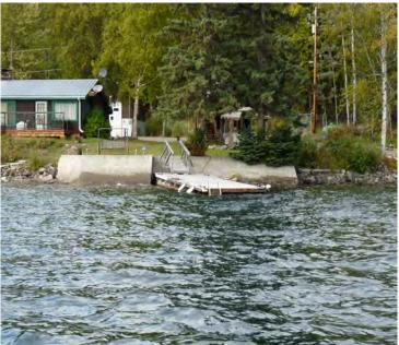
**Photo 8:** This photo shows a moorage, bank armouring, and associated substrate modification and riparian vegetation removal occurring in Segment 7 along the Horsefly Lake foreshore.
