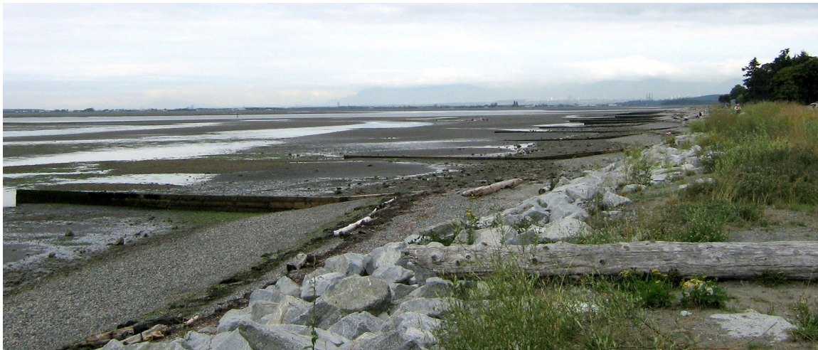
Figure 8: Shoreline hardening, Crescent Beach, Surrey, BC. An example of multiple groins, riprap armouring in the upper intertidal zone and foreshore dyking. Note the southerly flow of the drift cell as sediments accrete on the northern side of the groin. Photo Credit: R.C. de Graaf.
